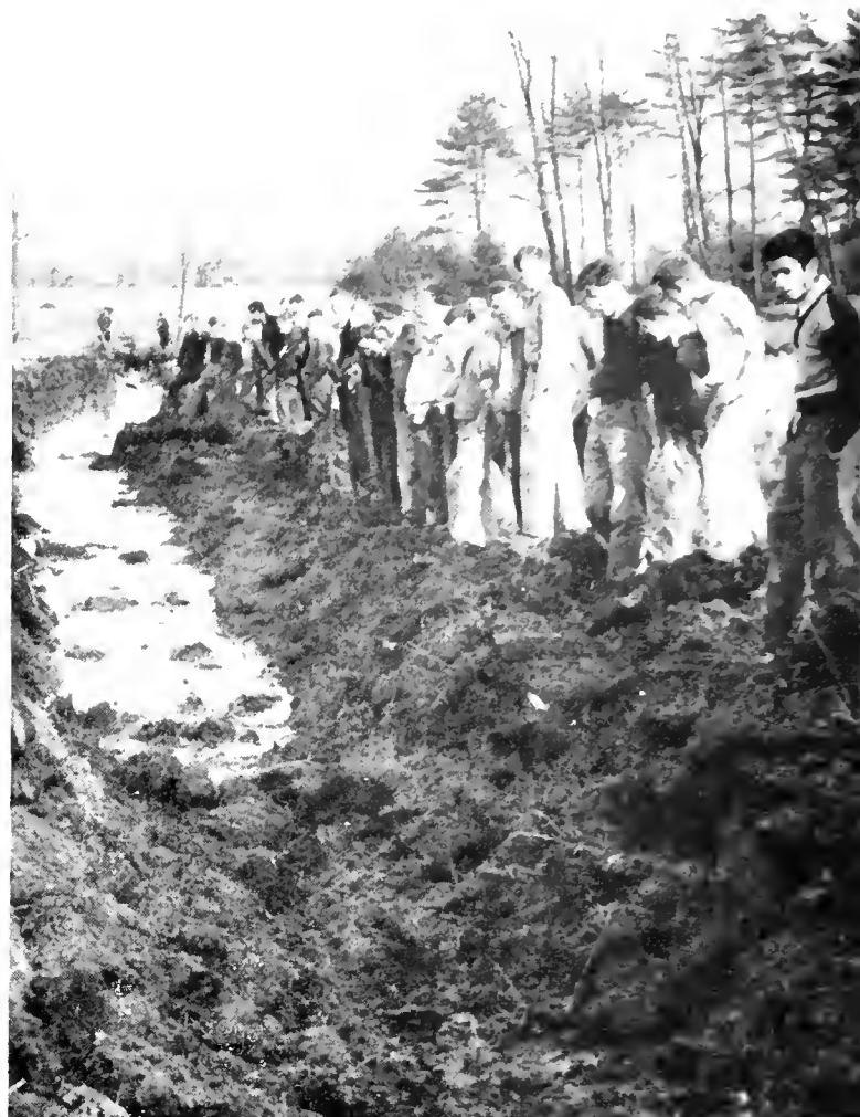
This is how the ditch looked when the class returned to inspect the results of the blasting. Students study and apply on their farms practical methods in farm mechanics.
